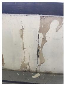
Water damaged drywall underneath sliding window
