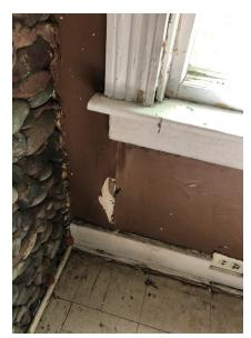
Bowing lintel in kitchen, with cracking plaster or drywall
