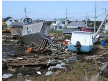
Damage from Hurricane Juan Storm Surge Photo Courtesy Chris Fogarty
