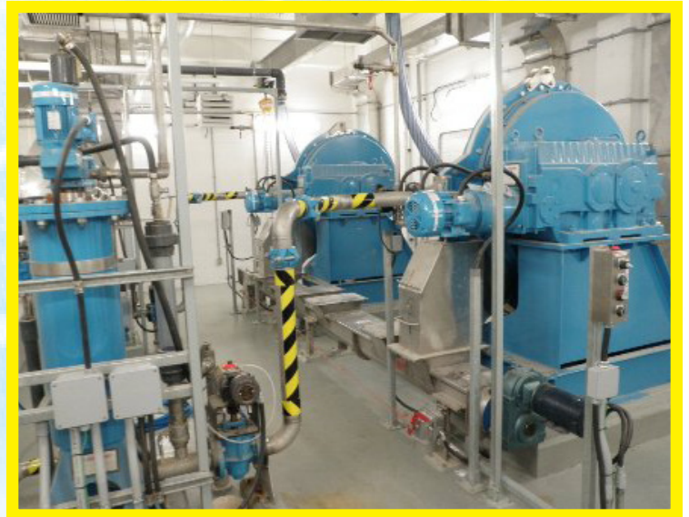
Herring Cove WWTF Press Room, March 2010
