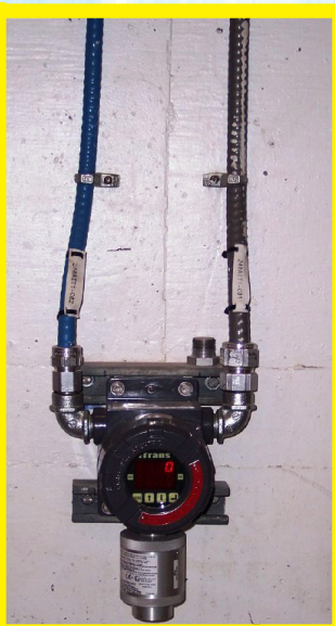
New gasmeters installed and commissioned in the Halifax WWTF, March 2010
