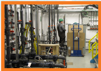
Crews working in Polymer feed area of Halifax WWTF
