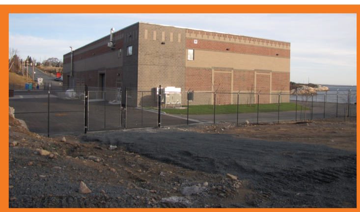
Herring Cove WWTF, October 2009.
