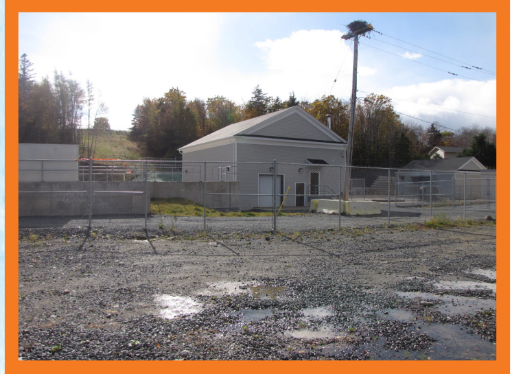
Environmental enhancements at Roaches Pond pumping station and Retention tank, October 2009.
