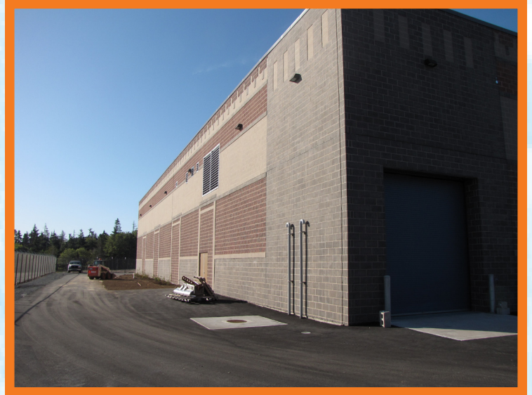
Herring Cove WWTF, September 2009
