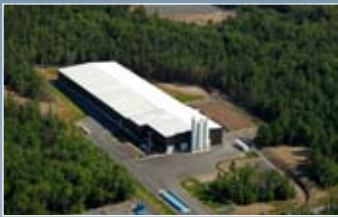
BioSolids Processing Facility, Aerotech Park, 2007
