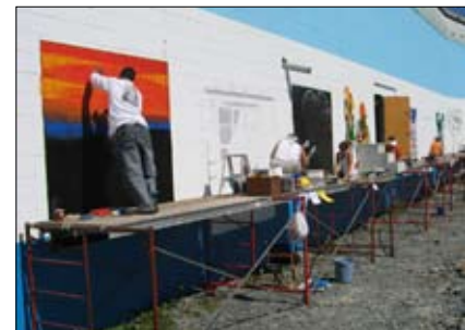
Reducing graffiti - community artists paint murals along the Harbour Front Trail, Downtown Dartmouth
