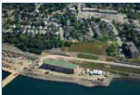
Harbour Solutions Project - Dartmouth Waste Water Treatment Facility
