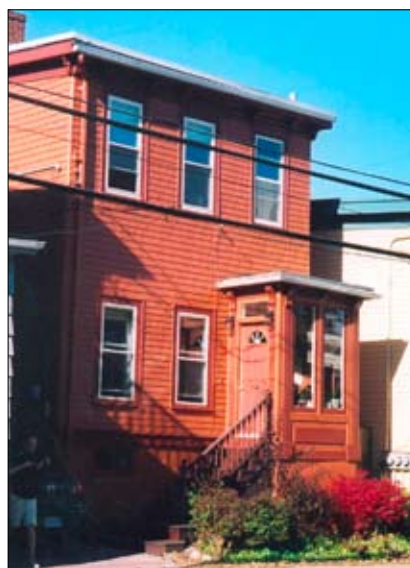
Registered heritage property, North Street, Halifax
