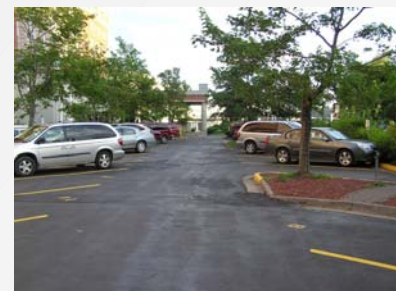
Appropriate landscaping can improve the aesthetics of parking lots and reduce stormwater run-off and urban heating.
