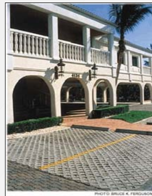
Permeable parking technologies can drastically reduce the stormwater runoff from parking lots.
