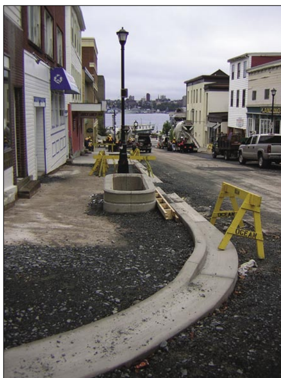
Portland Street Construction
