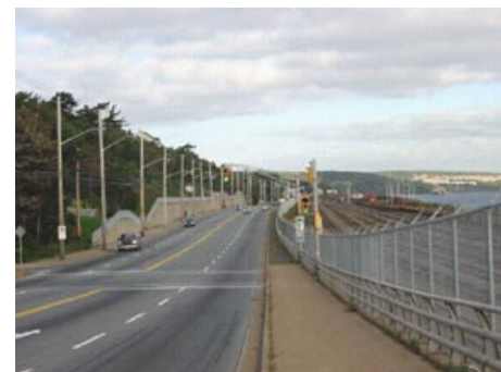
South of Bayview, Looking North 4 travel lanes, including two wide curb lanes provide adequate space for cyclists
