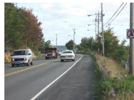
At Farmer Clems, Looking North Pave the shoulders 1.5m on both sides of the road.
