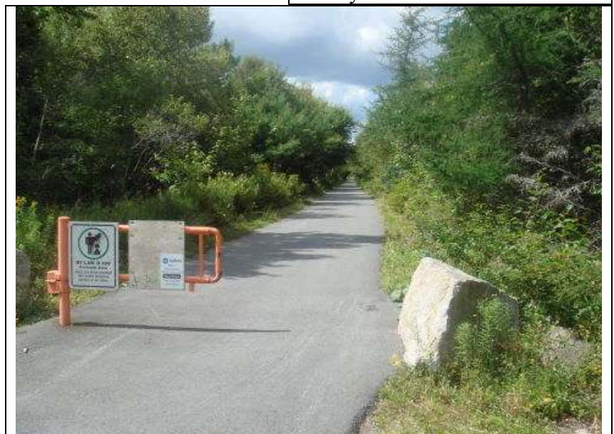
Example of a Paved Trail... (Part of the BLT Trail)
