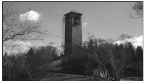
Memorial Tower Restoration
