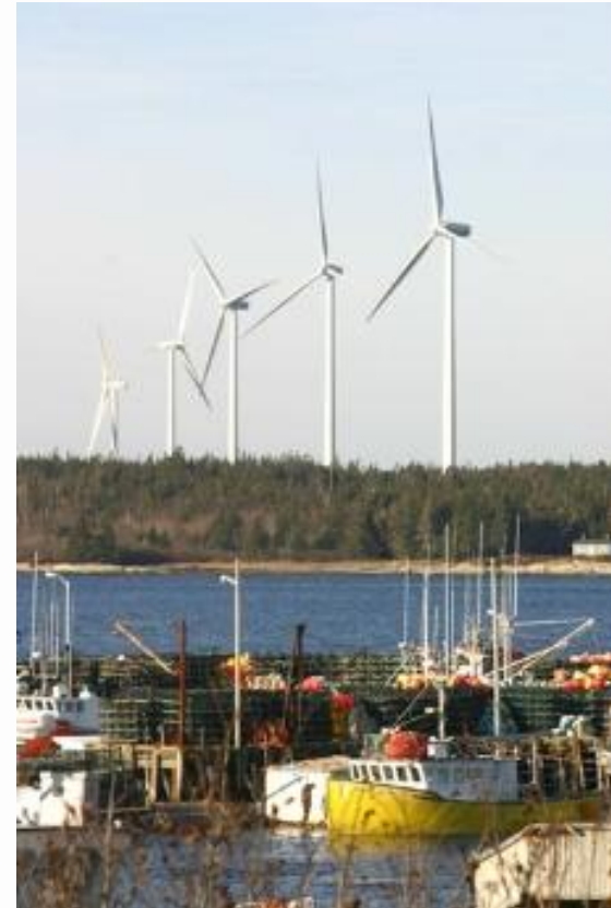
Wind farm in Pubnico, Nova Scotia Source: Chronicle Herald
