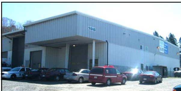
New Mechanical facility located at 196 Waverley Road, Dartmouth
