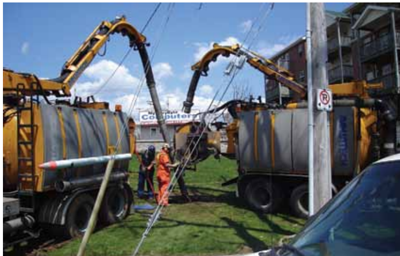
Sewer line cleaning, Northwest Arm, Halifax
