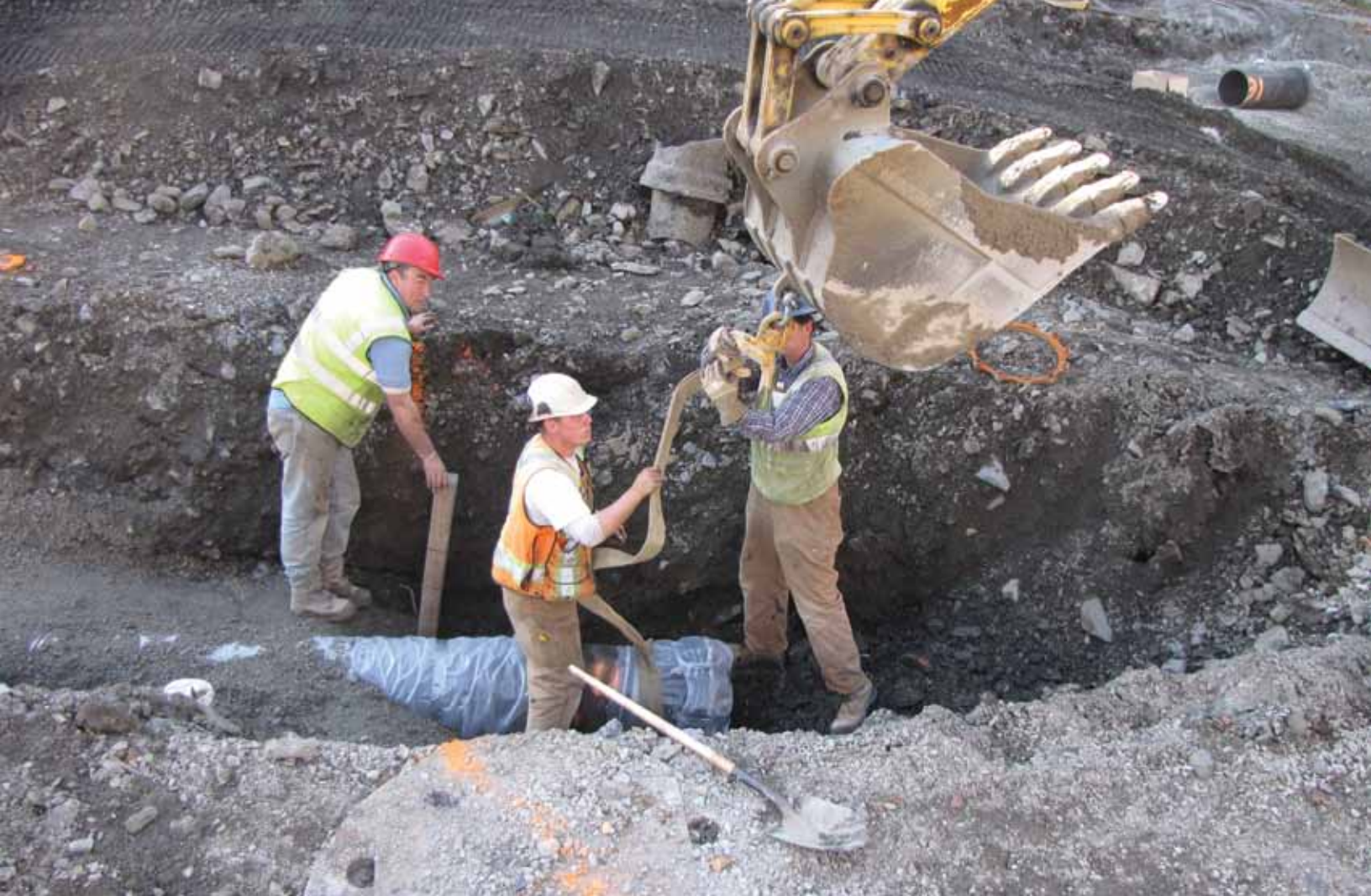
Above: Crews replace water line on South Park Street, Halifax
