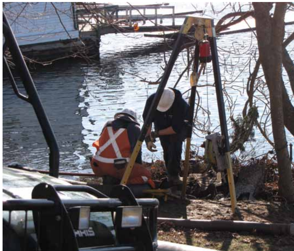
Sewer liner moving through leaking section of Northwest Arm pipe, Halifax
