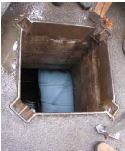
Sewer liner moving through leaking section of Northwest Arm pipe, Halifax
