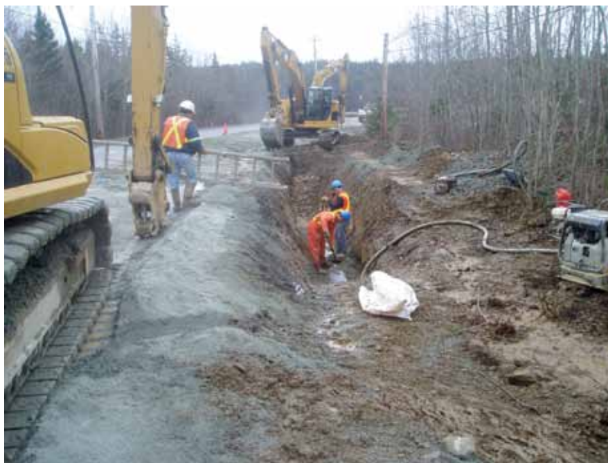
Service installation to the community of North Preston
