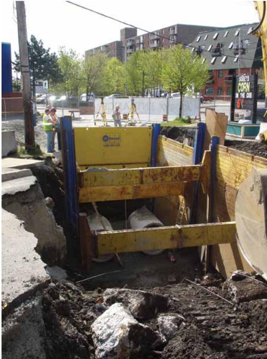
Freshwater Brook sewer replacement project
