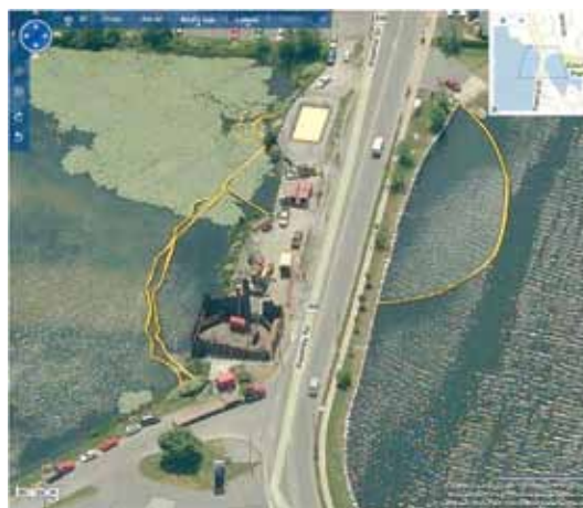
New wastewater pumping station at Red Bridge Pond, Waverley Road
