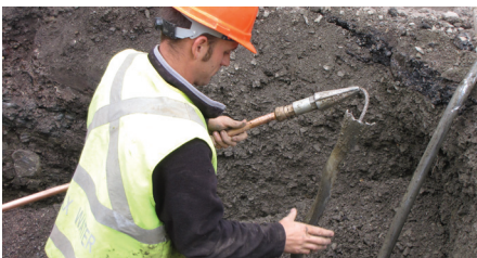
Installing a new copper line
