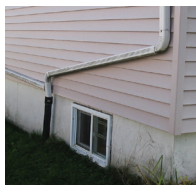
Improper Connection
