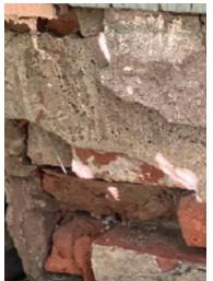
**Fig. 35** Foundation is structurally unsound, and will be replaced with a new foundation featuring reclaimed brick veneer.
