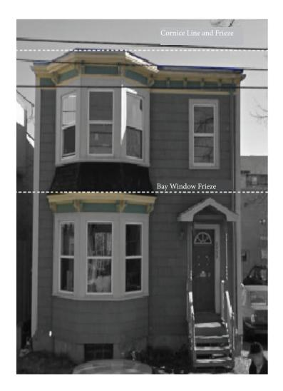
**Fig. 13** Horizontal elements showing characteristics of the Halifax Box style. The frieze features ornamental cornice brackets to accentuate the roof lines.
