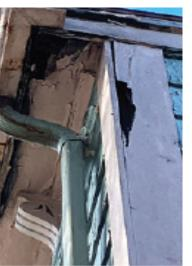
**Fig. 36** Soffits and corner boards will be repaired or replaced and repainted.
