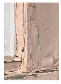
Fig. 34 The window trim is mostly rotten and will be replace. The vinyl Windows are outworn and will be replaced with triple glazed vinyl windows to look original
