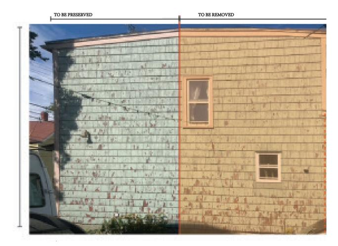
As the sides of the Halifax box form were normally never visible, keeping the majority of the house and restoring the front retains all key Heritage Defining Features. The joist structure of the house as drawn on page 27 makes the proposed removal fairly simple. As stated, the alternative to this would have been the complete demolition to make room for a conventional development.
