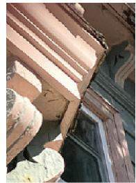
**Fig. 33** Wood work will be scraped and repainted if not rotten or replaced using the original patterns.
