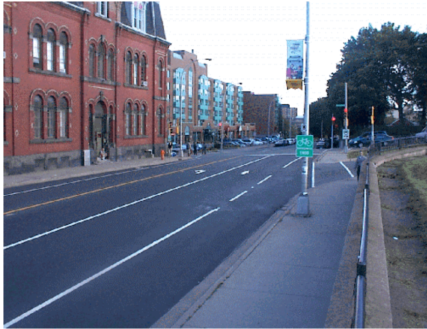
Fig.11: Southbound cycle lane on Brunswick Street at the Sackville Street right hand turn off. The skip lines begin at the turn off rather than in advance of it as recommended by design guidelines.
