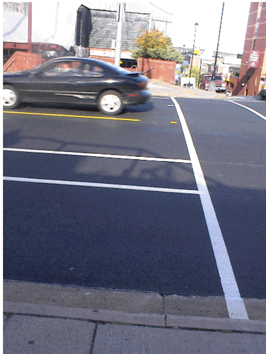
Fig. 7: Shown is the cycle lane meeting the crosswalk as recommended by design guidelines.
