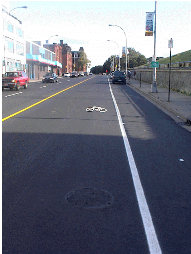
Fig. 9: Existing design of cycle route between George and Prince on Brunswick Street. There is no dedicated cycle lane. Bicycle icons replace the dedicated cycle lane existing on other segments of the cycle route.
