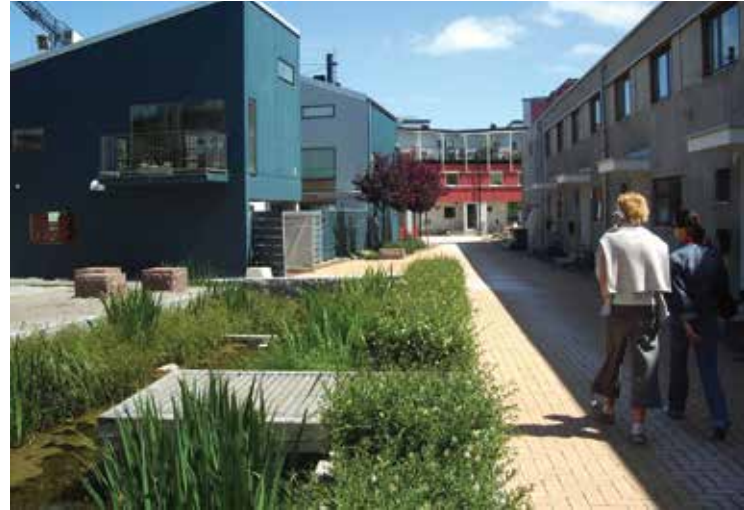
Stormwater Bioswale
