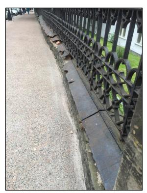
Figure 12: Bowed wall section & broken metal wall cap.
