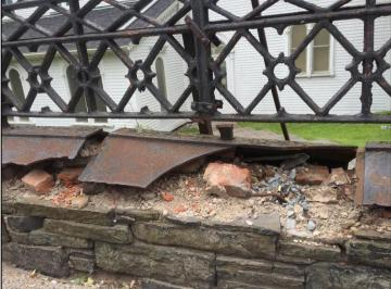
Figure 13: Failed metal cap and brick top course.
