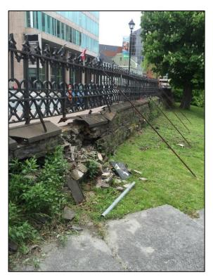
Figure 11: Failed wall section on Argyle Street.
