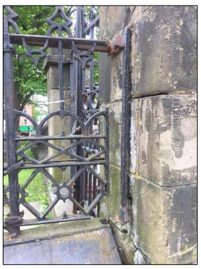
Figure 10: Ironwork failing at the Prince Street gates.
