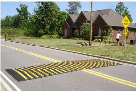
Sample of a speed hump used for traffic calming
