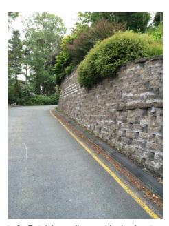
Photo 3: Retaining wall around bedrock outcrop.
