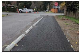
Figure 6: Temporary Sidewalk Installation in Seattle, Washington
