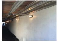
Figure 5 – Solid construction hoarding provides pedestrian protection from vehicles, overhead objects, and provides physical separation from the site activities. Lighting for covered ways is an important consideration.
