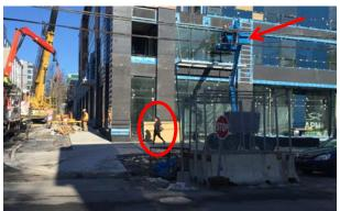
Figure 4 – Without appropriate site controls in place pedestrians are forced to cross streets at unsafe locations or pass directly through an unprotected work area and even underneath active equipment.
