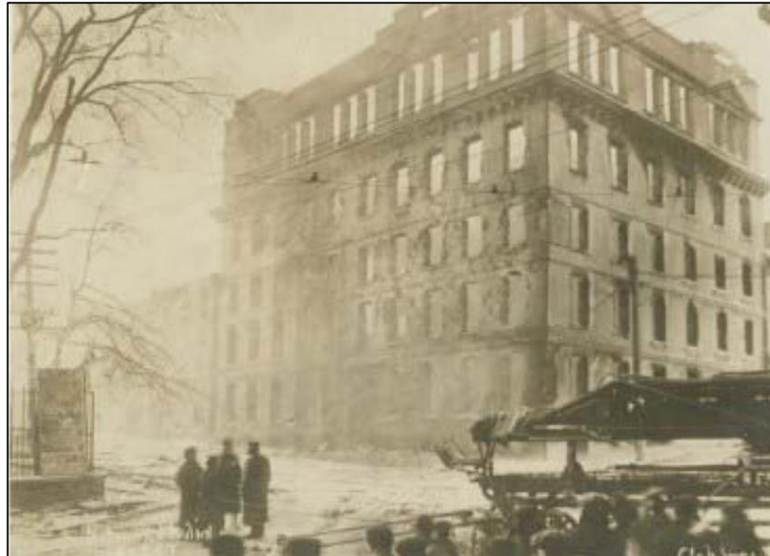
The Kenny-Dennis building showing the shell of the four-storey granite façade topped by the one-storey 1901 addition, shortly after the fire in 1912. Source:
