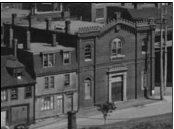
Figure 4: Photograph showing the Salvation Army Citadel, 1900. Note the chimneys, finial ornament, and ornamental parapet along the roof line (Source: LAC).
