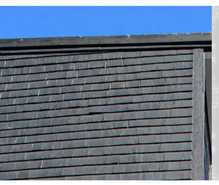
West elevation: deteriorated wood singles, cupping cracking and lifting
