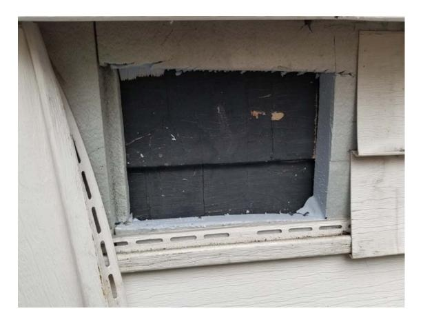
Based on inspection of sills around the building, this insulation layer exists around the building.
