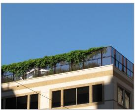
Image 3 - Examples of Porous Parapets
