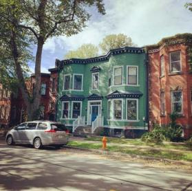
Figure 6: The white vinyl siding (Left: Google Street View 2016) was removed in 2018 and the building façade was rehabilitated with wooden shingles (Right: Google Street View 2018)
