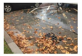
Figure 7 – Porous asphalt in Halifax; water can infiltrate through the asphalt, but sediment may be trapped.
