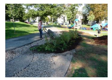
Figure 4 - A rain garden being constructed outside the George Dixon Center in Halifax, with the help of the Ecology Action Center
