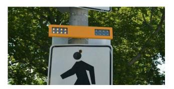
RRFBs are pedestrian activated crosswalk systems which consist of two rapidly and alternately flashing rectangular amber beacons mounted above the side mounted pedestrian crossing signs. RRFBs can enhance safety at unsignalized intersections and mid-block pedestrian crossings by increasing driver awareness of potential pedestrian conflicts and by improving driver yielding behavior.
