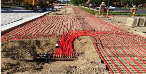
Typical Snowmelt Tubing Manifold
