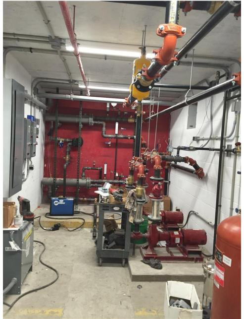
Typical snowmelt system mechanical room with heat exchangers and pumps
