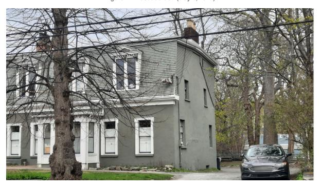
Figure 12: Evidence of original gable roofline on the west facade (May 4, 2021)
