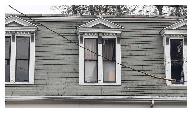
Figure 8: Dormers with pediment style roof, dentils and corbels (May 4, 2021)
