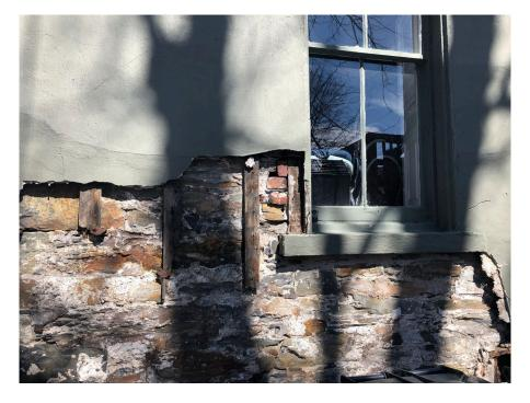
Figure 10: Evidence of original rubble stone walls underneath stucco cladding on south façade (April 9, 2021)
