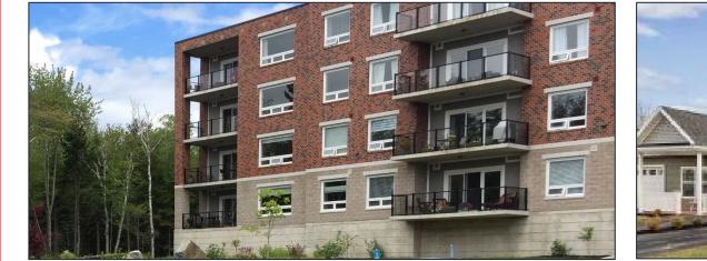
Multi-unit residential building with small casement windows that are easily accessible from interior of units. First floor are raised to improve safety and security
