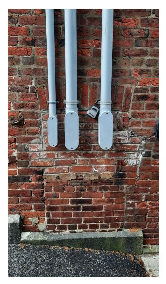
Figure 24: Blinded window on the south elevation (July 17, 2021)
