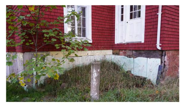
Figure 25: Detail view of foundation damage to northwestern corner of 144 Pleasant Street (October 19, 2021)
