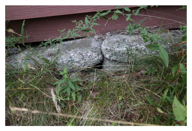
The footing is also not continuous. There are sections where the building appears to be resting on the ground.
