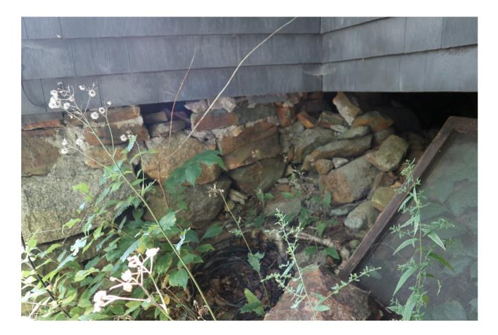
As is obvious in these photographs, what is there would no longer qualify as a secure foundation. It is now more along the line of a building being supported by piles of rock. There is one corner of the building which is actually supported by a few stacked concrete blocks. This is clearly shown in the photograph on the previous page.
