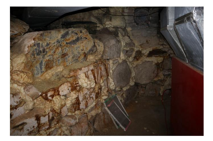
Water entering the building can and has done a lot of damage to electrical wiring and mechanical equipment. There is visible evidence of rot on post and beams within the basement area. Earlier is was pointed out the condition of the exterior of the wood wall to top of these foundations. Basically everything which is in contact with the ground or these rock wall has rot and mold on it to some degree.
