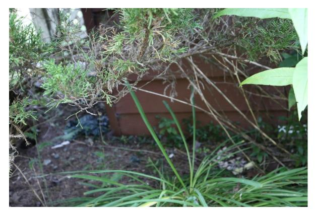
Compounding this improper condition, there is a good portion of the building exterior wall in which the wood siding is at or near the grade line. This can and probably has led to water infiltration into the building. Visible evidence of this is in the rot and possible mold along the lower coursed of wood siding.
