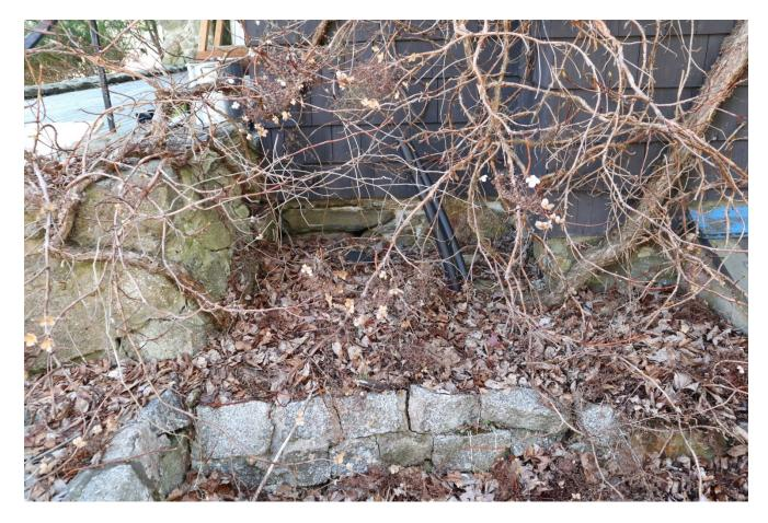
Around the building there are a number of rock walls. Some of these are for the support of rock stairs, others to support deck areas, and others simple as architectural features. In all cases you can clearly pick out the fact that these wall have failed.
