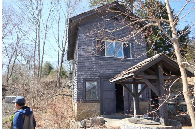
2) The windows in this building are not in good condition. Most are wood frame single pane glass. These have a significant amount of rot and are in bad need of paint, repair or replacement.
