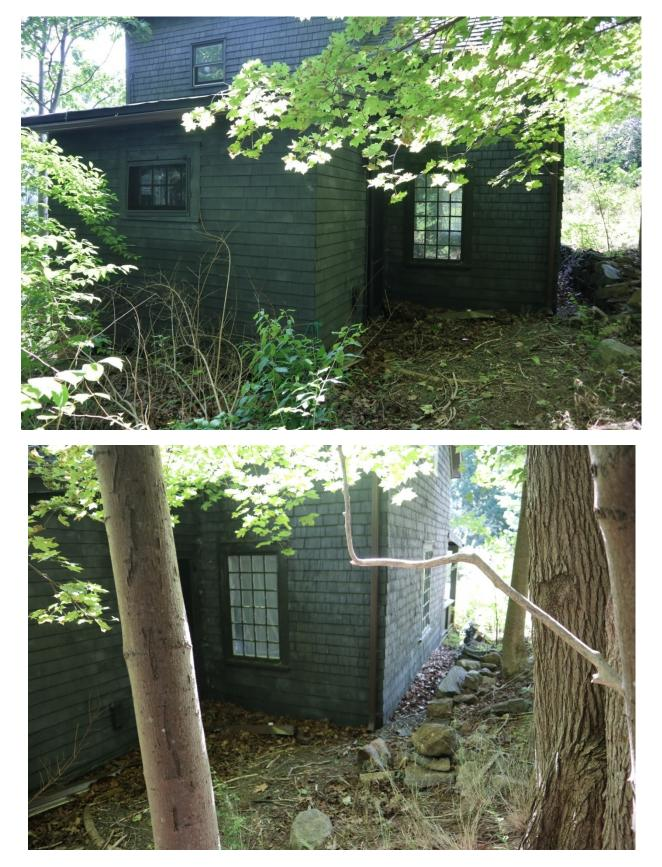
Compounding this improper problem, was the fact that a good portion of the building exterior walls have the wood siding at or near the grade line. This has led to rot of the siding and the wood wall structure, and water infiltration below building. The space below the building is basically a crawl space.
