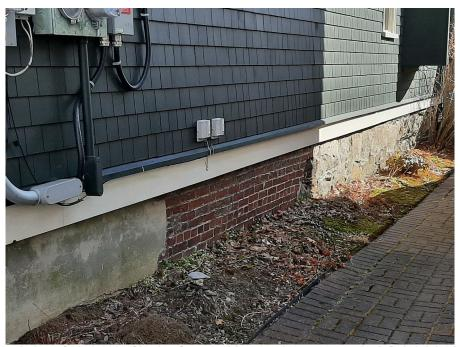
Figure 12: Foundation of 6032-6034 Charles Street, with parged concrete to the left, brick in the centre, and rubblestone and granite blocks to the right (Staff photo, 22 February 2023)
