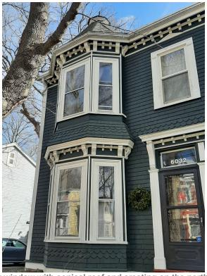
Figure 13: Two-storey Bay window with conical roof and cresting on the north elevation (Staff photo, 22 February 2023)
