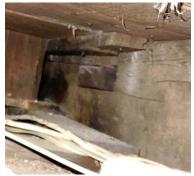
Figure 3: Photo showing the subject dwelling's timber frame construction with a mortise and tenon joint.
