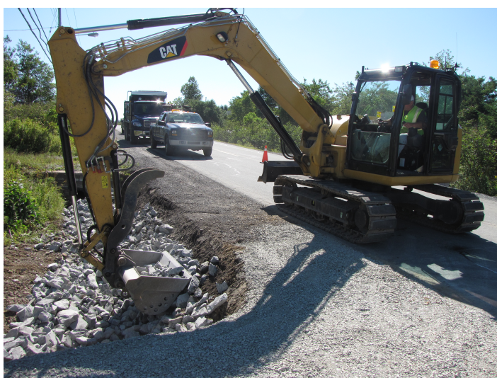
Repairing and upgrading ditches to improve stormwater service.
