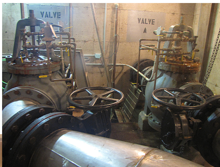
Orchard Control-Pressure Reducing Valve Chamber
