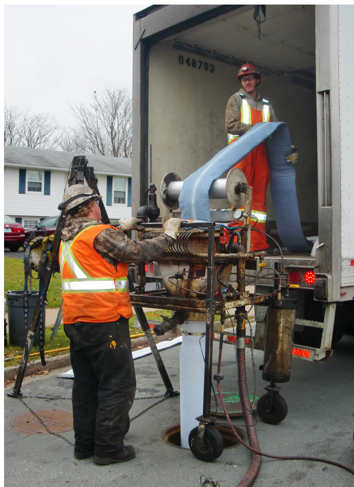
Sliplining - A cost effective, non-disruptive way to restore pipes.
