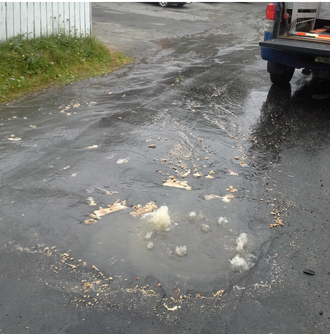
Sewer backup onto the street. A potential public and environmental health risk.
