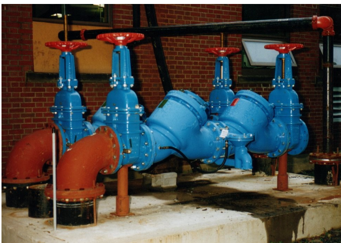
Installation of a backflow preventer at a local hospital
