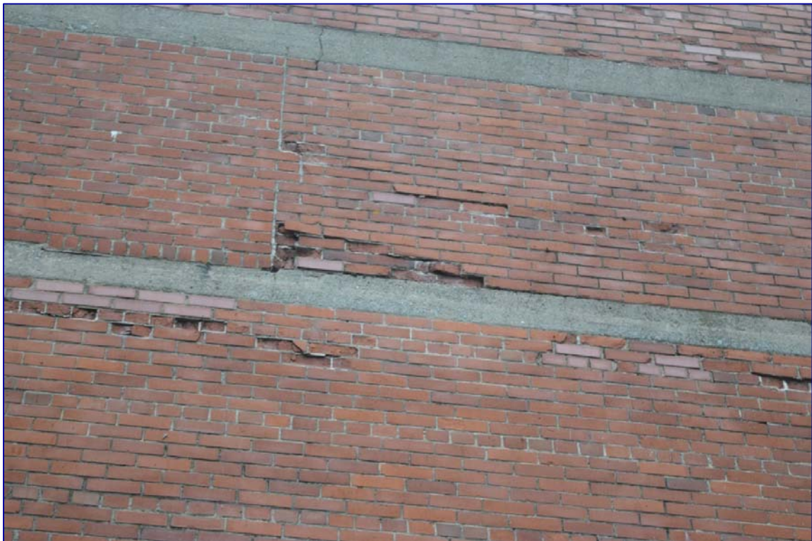
Image from the south elevation of the Forum taken October 2017
