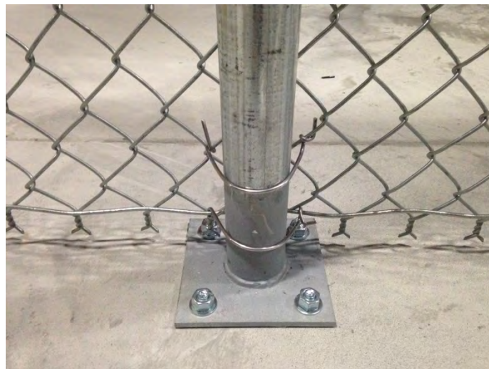
Figure 1: Rigid Fence Fixed to Concrete Sidewalk
