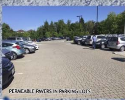
PERMEABLE PAVERS IN PARKING LOTS
