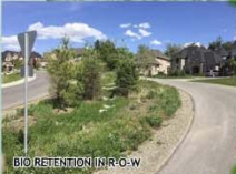
BIO RETENTION IN R.O.W
