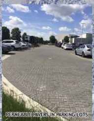
PERMEABLE PAVERS IN PARKING LOTS
