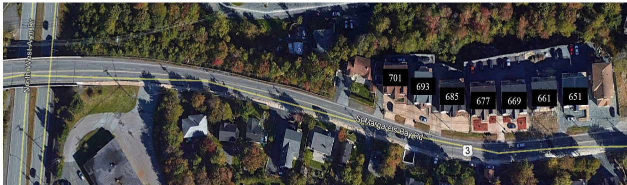
Figure 1A - Cornerstone Developments Limited apartment development 651 to 701 St. Margarets Bay Road
