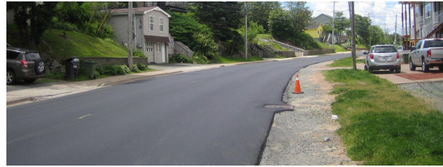
Photo 2A - Looking west on St. Margarets Bay Road towards the North West Arm Drive overpass from the shared driveway for 651 and 661 St. Margarets Bay Road.
