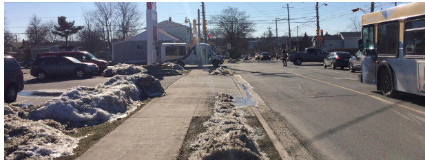
Photo 4 - Looking west on Albro Lake Road towards Victoria Road intersection from an existing site driveway.
