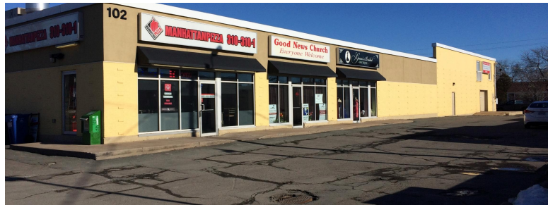
Photo 1 - The front of the building as seen from the Albro Lake Road driveway. The motor vehicle service centre will occupy the right (south) end of the building.
