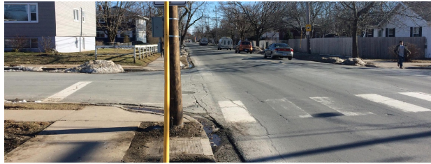
Photo 2 - Looking south on Victoria Road towards Chappell Street intersection from an existing site driveway.
