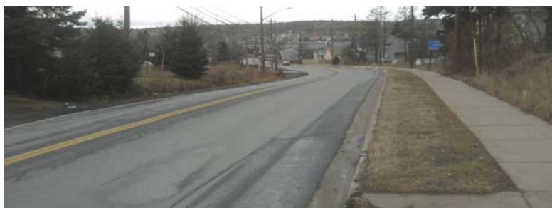
Photo 2 - Looking west on St. Margaret's Bay Road from the proposed new street intersection.
